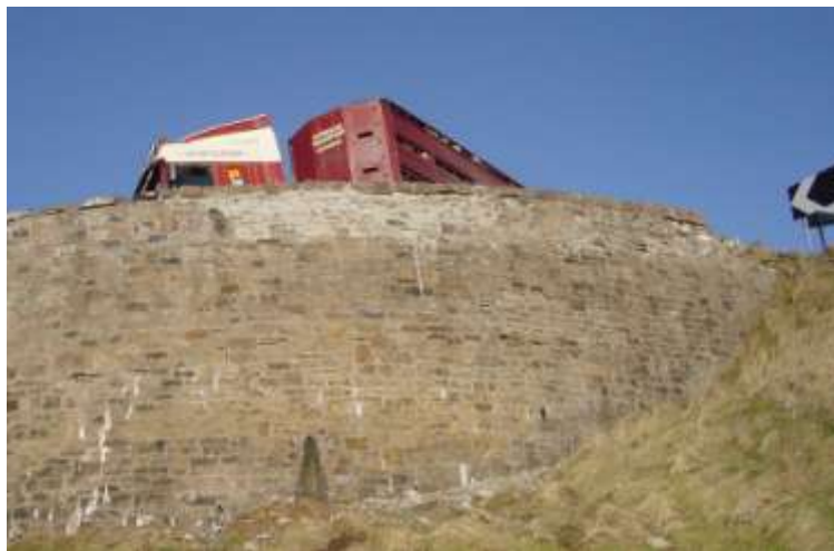
Fig 9 4m high retaining wall below North Hairpin Bend
