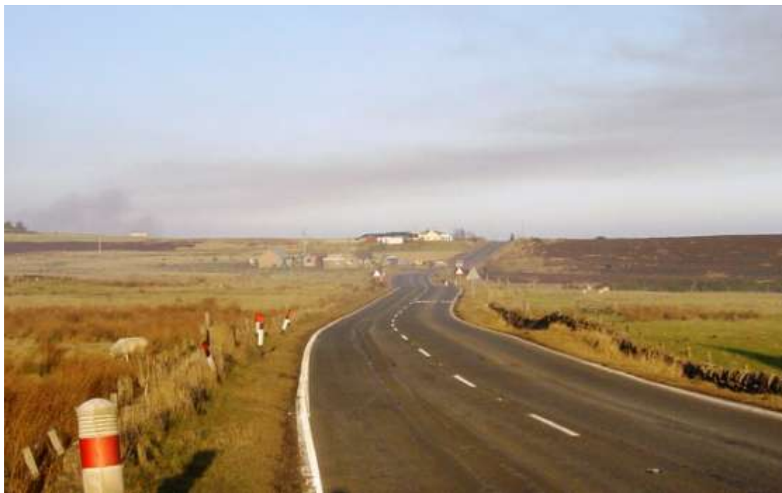
Fig 16 Ramsraigs. Good visibility but a minor narrow bridge prevents overtaking
