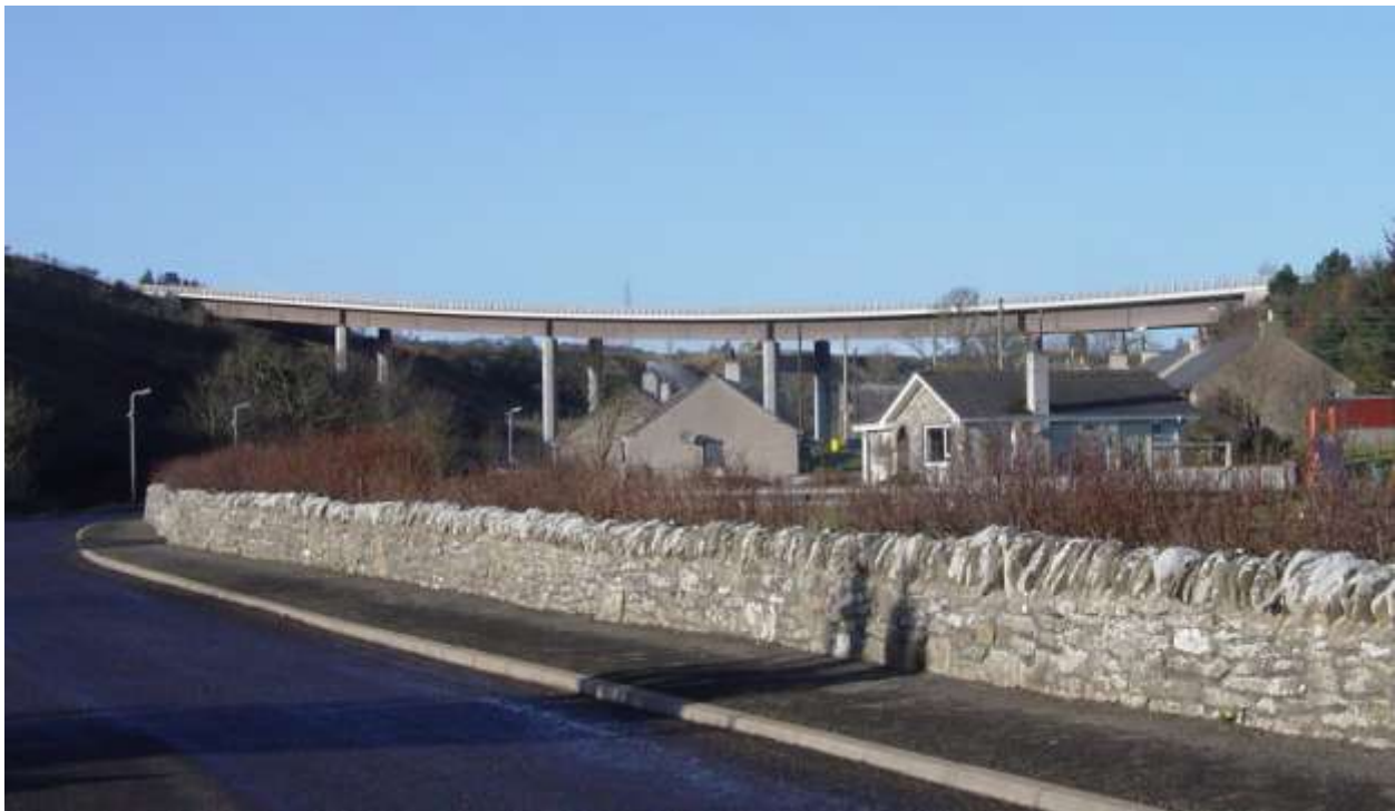
Fig 8 Dunbeath viaduct. Viaducts at Berriedale would be very much longer and higher
