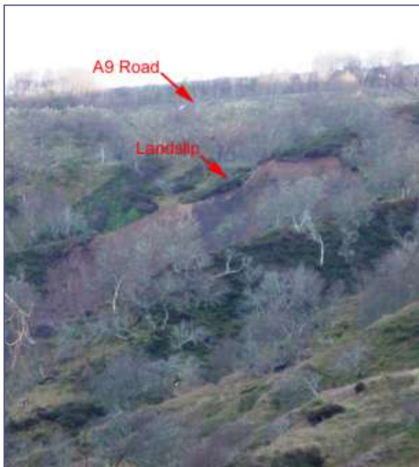
Fig 2 Landslip below A9
