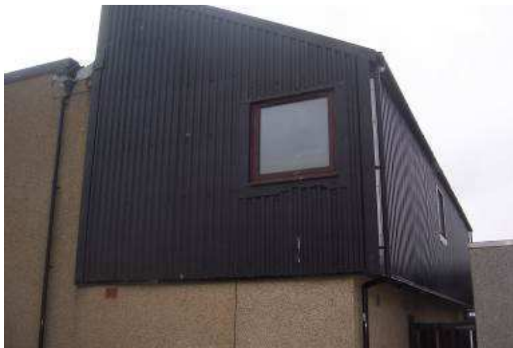
View looking at SE corner
