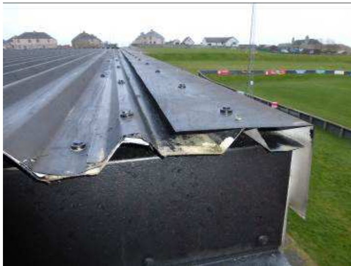
Squash court verge flashing at box gutter external corner
