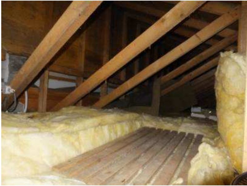
Pitched roof void looking at vertical abutment
