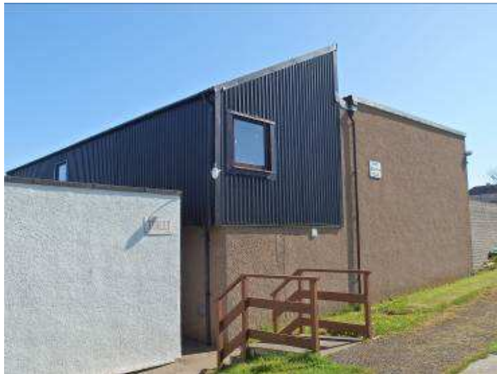
View looking NE
