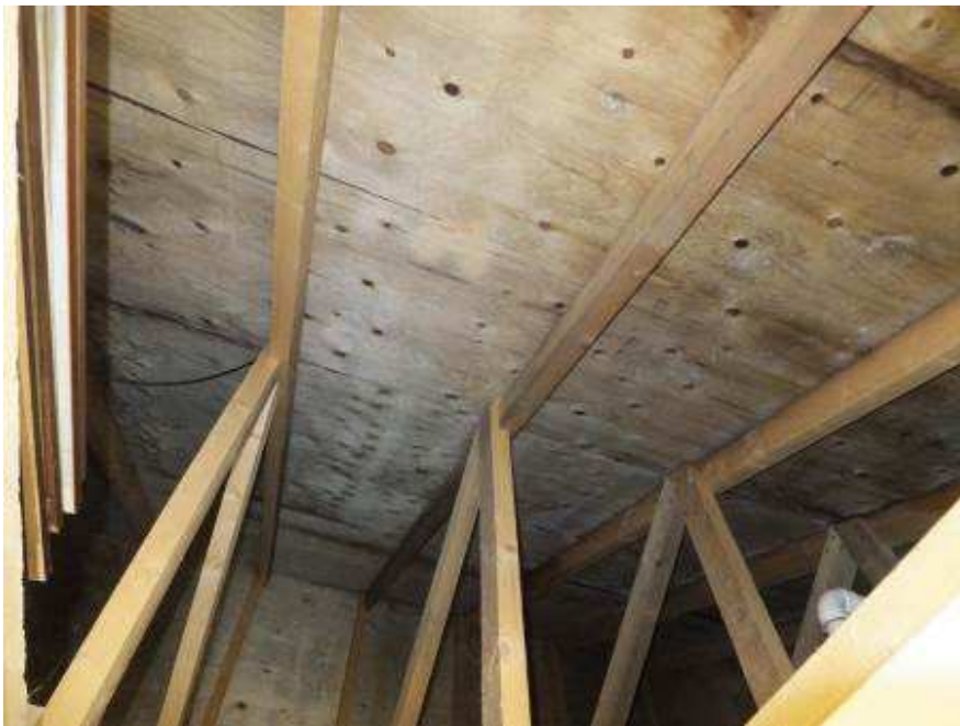
Pitched roof void looking at sarking
