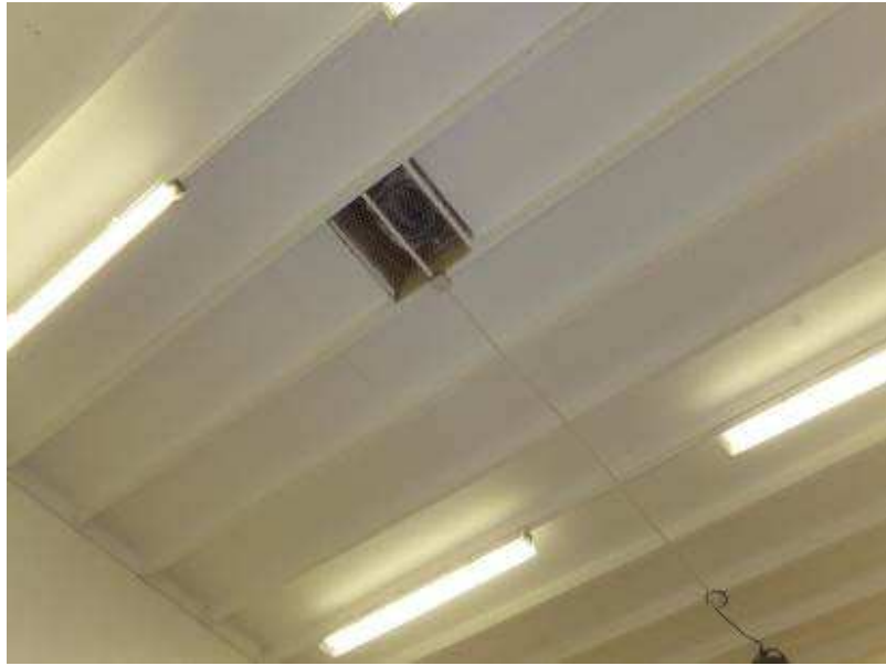
Squash court ply box beams
