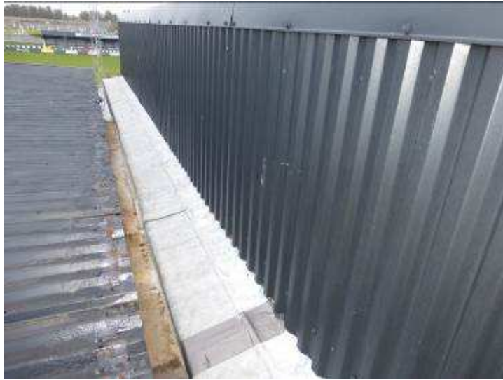
View looking at vertical abutment & gutter details
