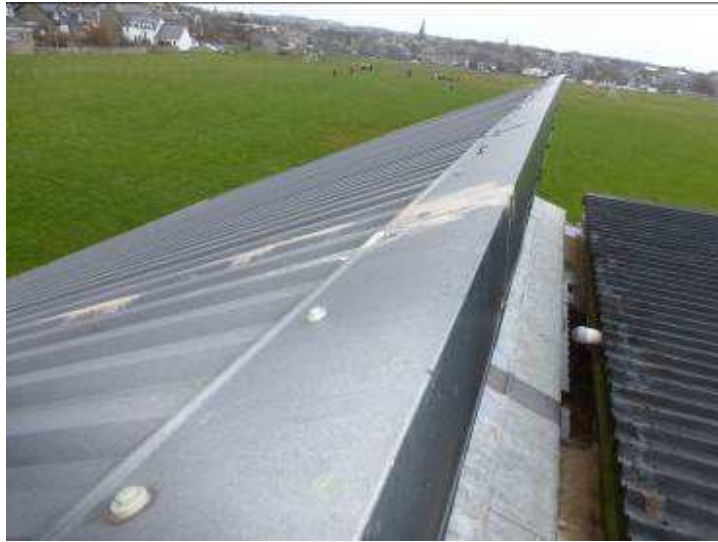
Mono ridge flashing
