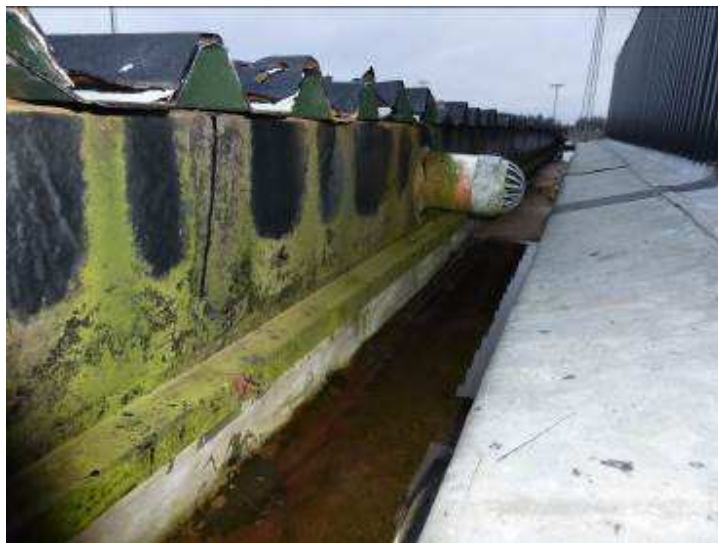
Box gutter detail
