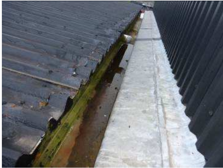
Box gutter view
